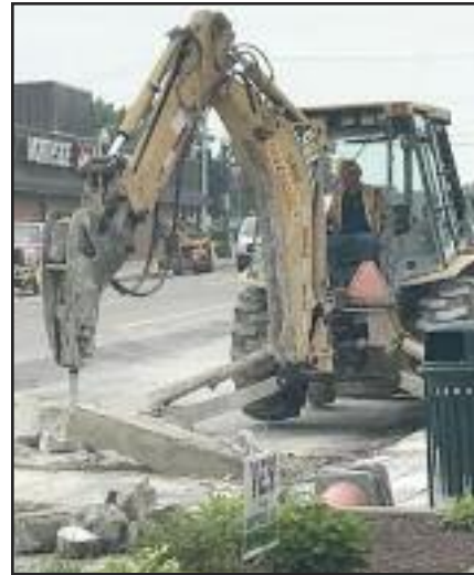
Construction of Wayne Road is scheduled to be complete by November. Photo by Maxwell Cameron
